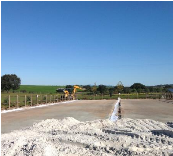
Simplified drainage system with additional drainage ditch
