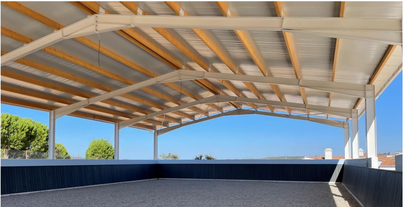
Roofing with sandwich steel plates with wooden purling's
